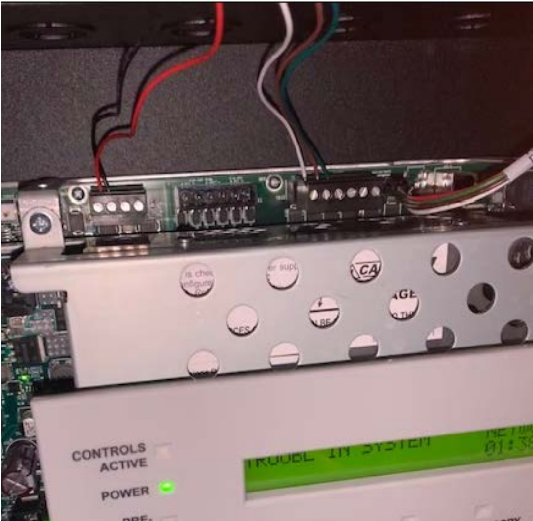
640/320 Power and Printer Port Connections
